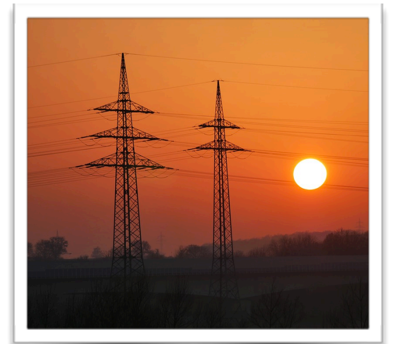
Access to electricity
